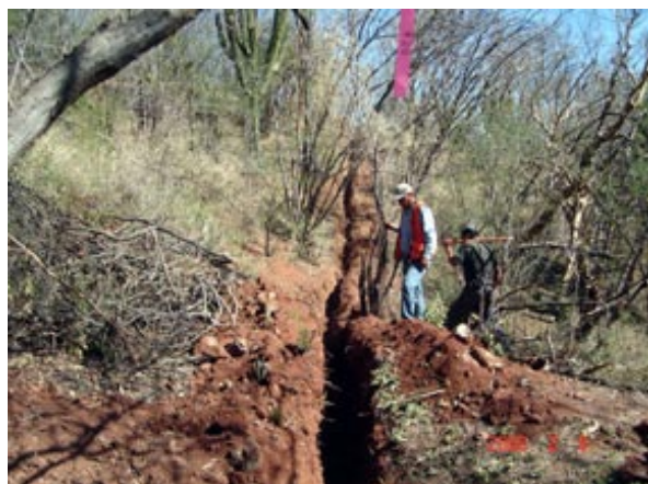
Trenching at the Carol Property
